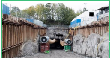
Grouting from ground surface and tunnel entrance
